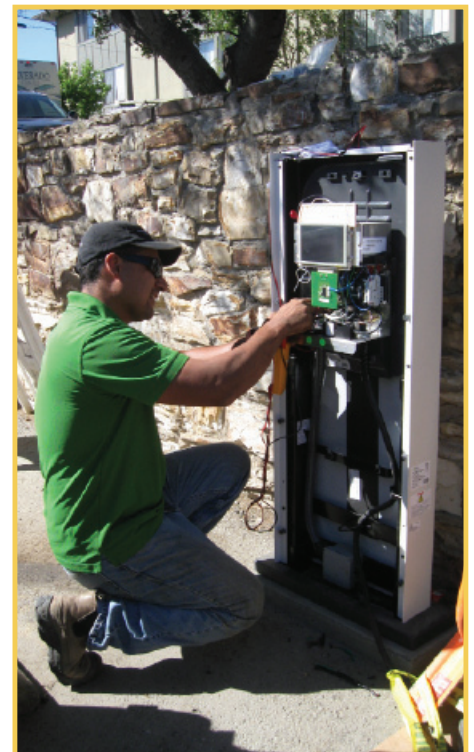
Figure 12. Station Installation. Gabriel of Regalado Electric installing the Blink Station at the Sunset Center in Carmel.
